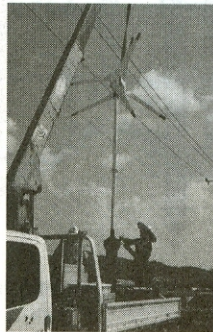
Figure 1. Operating test of the counter rotating wind turbine using vehicle
